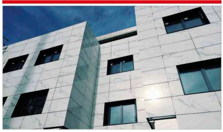
Isotec Parete has been fixed directly on the prefabricated infill panels in reinforced concrete. The 60 x 120 mm ceramic slabs have been anchored to the Isotec Parete steel stiffener by means of a special mechanical anchor in patented steel, which is inserted in the kerf cut on the thickness of the ceramic to create an attractive concealed effect. The final result is an energy-efficient building of great appeal, characterised by an original and elegant finish.
