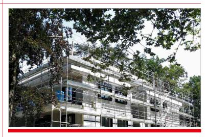
The structure of this new building, characterised by a geometric and linear architecture, is entirely in reinforced concrete and has been completely insulated with ventilated façades made of 160 mm thick lsotec Parete panels; for the external cladding has been chosen a ceramic white "Calacatta" marble glossy finish, for a very elegant effect, for a total surface area of 700 sqm.
